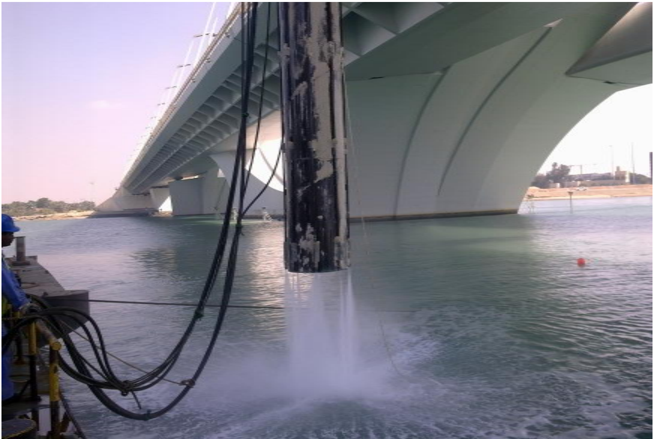
Figure 7. Water Jet Method - Casing Pile.
