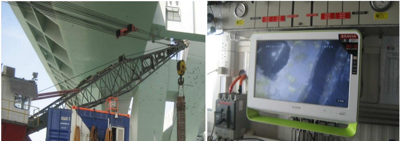
Figure 13. Casing Pile positioning inside an Existing Pile and view from the Diver's Screen.
