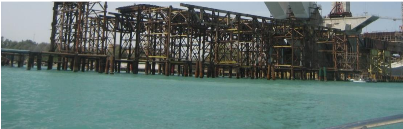
Figure 1. Temporary works – Falsework Erection on Piles.
