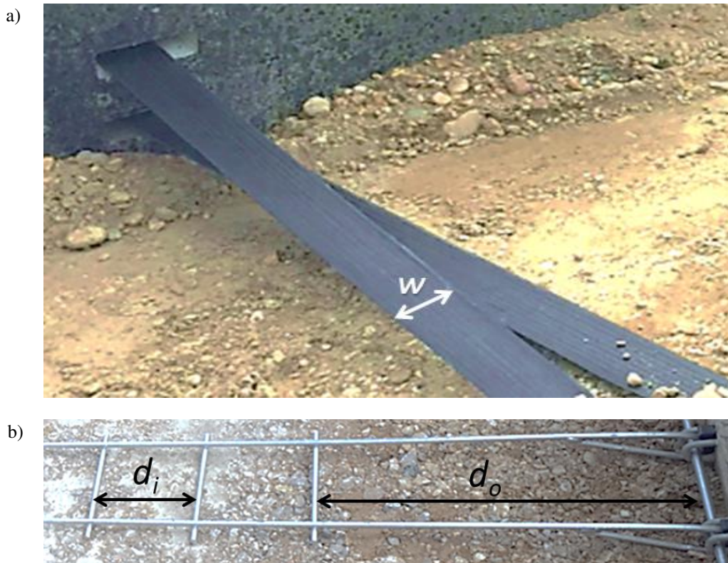
Figure 2. Details of the VSOL® wall reinforcement types used in the D4R7 Project: (a) polymeric strips and (b) galvanized steel ladders and related connection systems (void formed and clevis loops, respectively).
