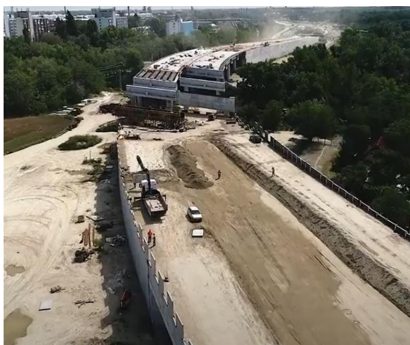
Figure 4. Back-to-back D4R7 reinforced soil walls during construction.
