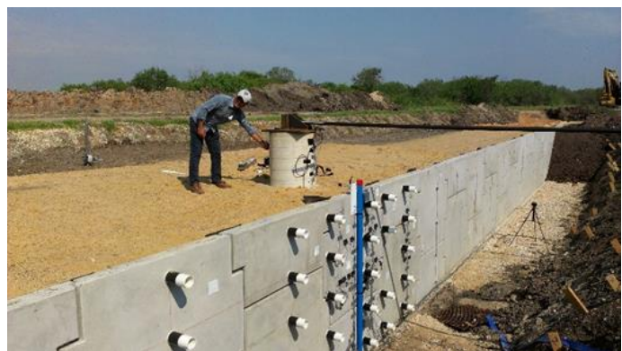
Figure 30. Construction of the MSE wall.
