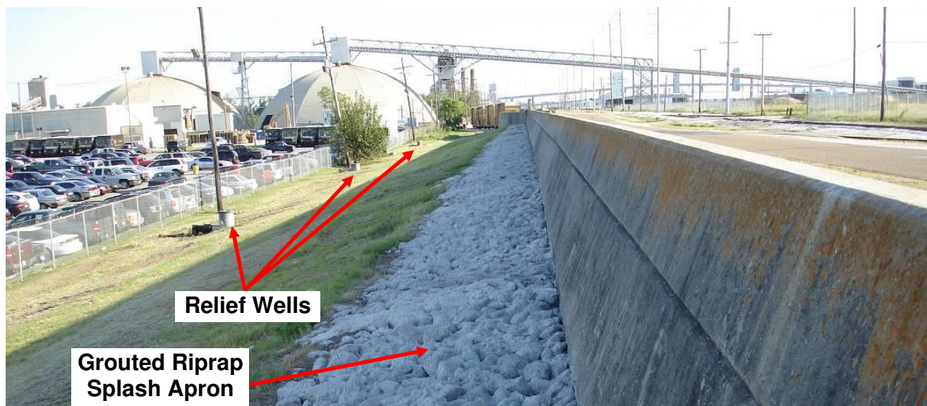
Figure 28. IHNC floodwall near East Morrison Road. Note splash apron (center) and relief wells (left). (October 2, 2008, 30.0248° N, 90.0295° W)
