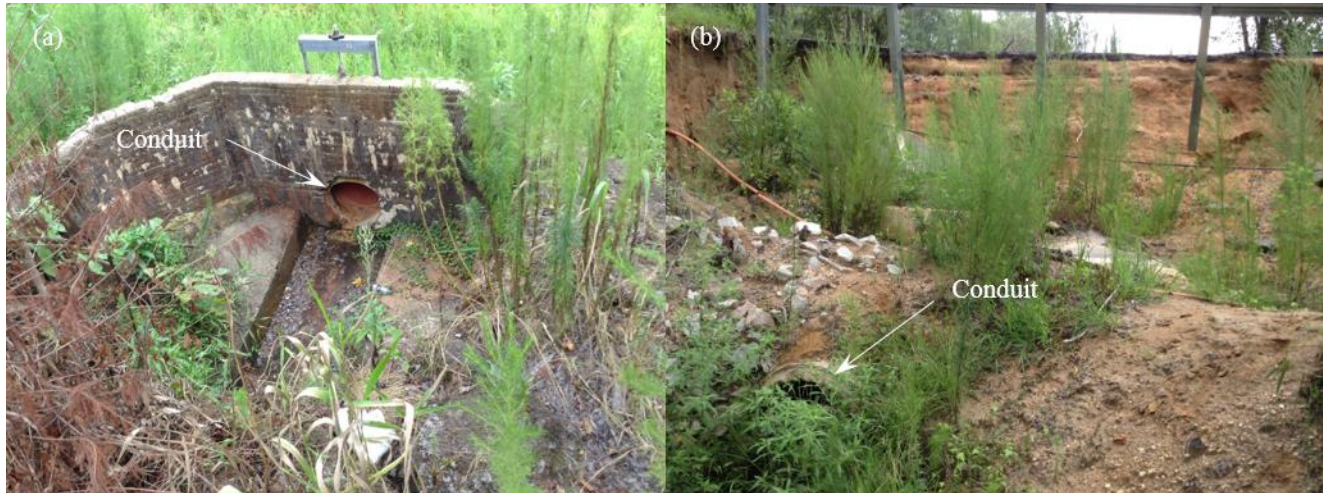
Figure 4. Spillway structure for Dam A: (a) conduit on upstream side (north view from SR-40-67), and (b) conduit and washed out soil above on downstream side (north view from downstream).
