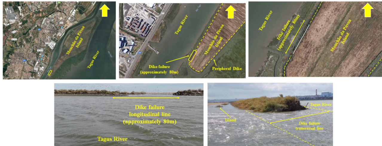
Figure 38. Location and view of the dike failure.
