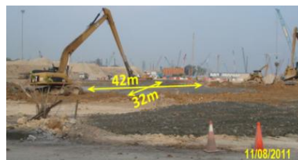
(d) Photograph of pond D (42 m x 32 m x 5.5 m) with slurry clay heaved from RL96.5 m to RL102 m.
