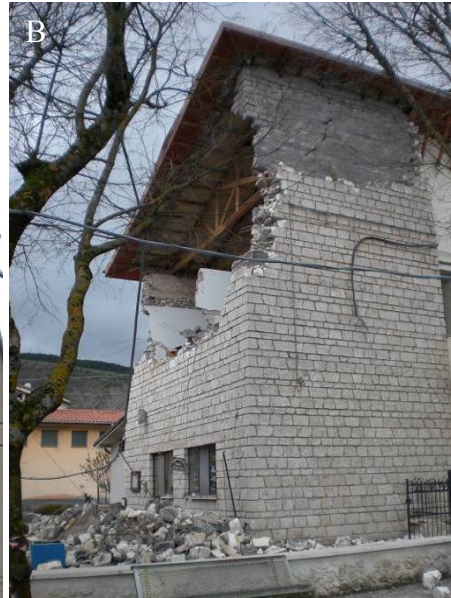
Figure 98. Goriano Sicoli. (A) Diagonal cracks in a masonry building (D3, (B) Partially collapsed masonry school (D4).
