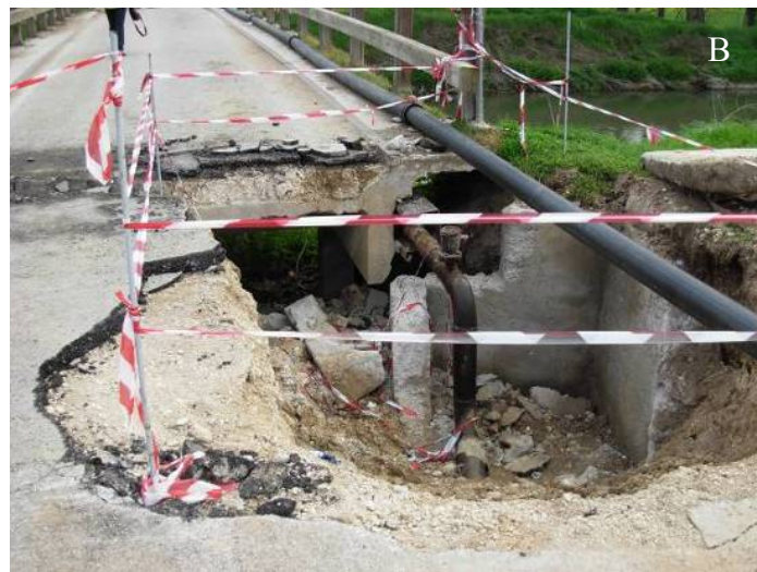
Figure 68. Onna. (B) Intense damage (D4) of RC bridges on the Aterno river.
