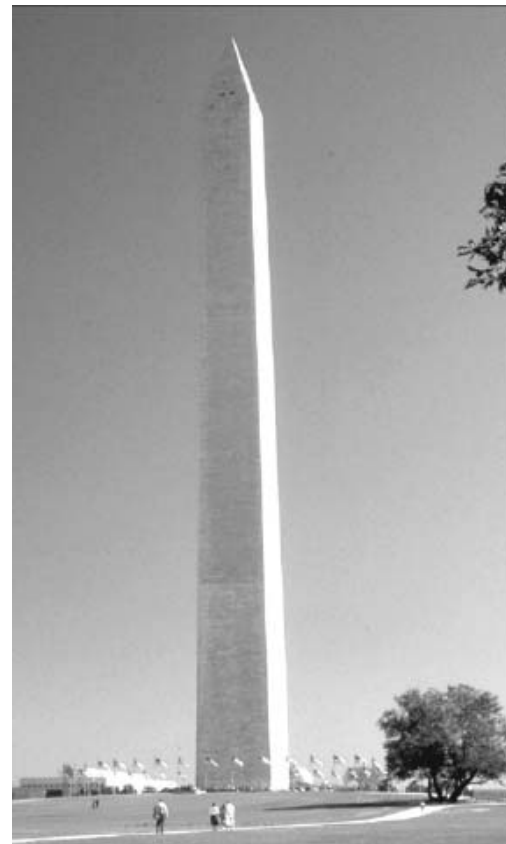
Figure 2b. Final design – constructed monument.
