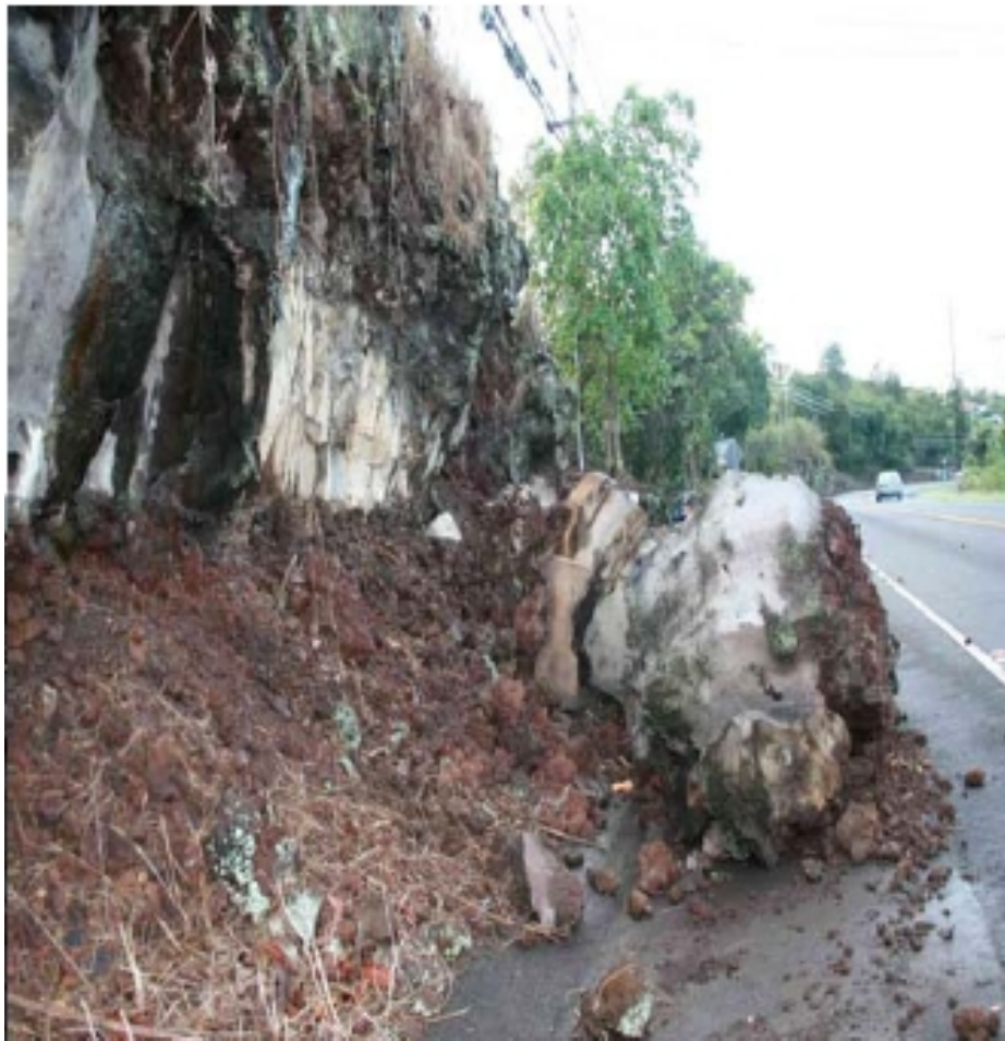
Figure 8. Failed rock cut: massive a'ā block undermined by raveled a'ā clinker (Chock, 2006; after Robertson et al, 2006).
