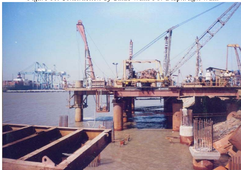
Figure 11. Construction of Piles.
