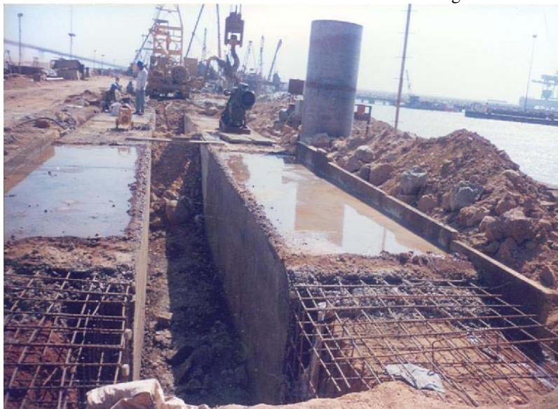
Figure 10. Construction Of Guide Walls For Diaphragm Wall.
